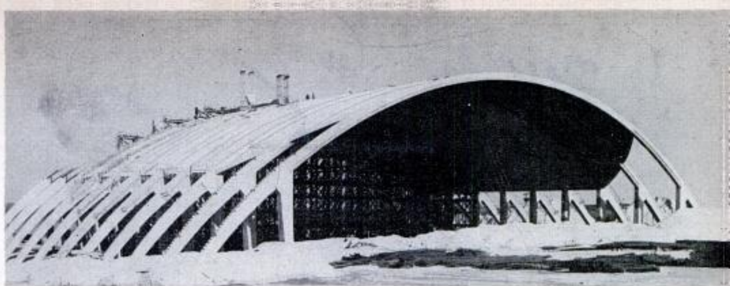
Interior scaffolds moved along on tracks as ribs were mounted and roof was laid. Arches at rear are unfinished
